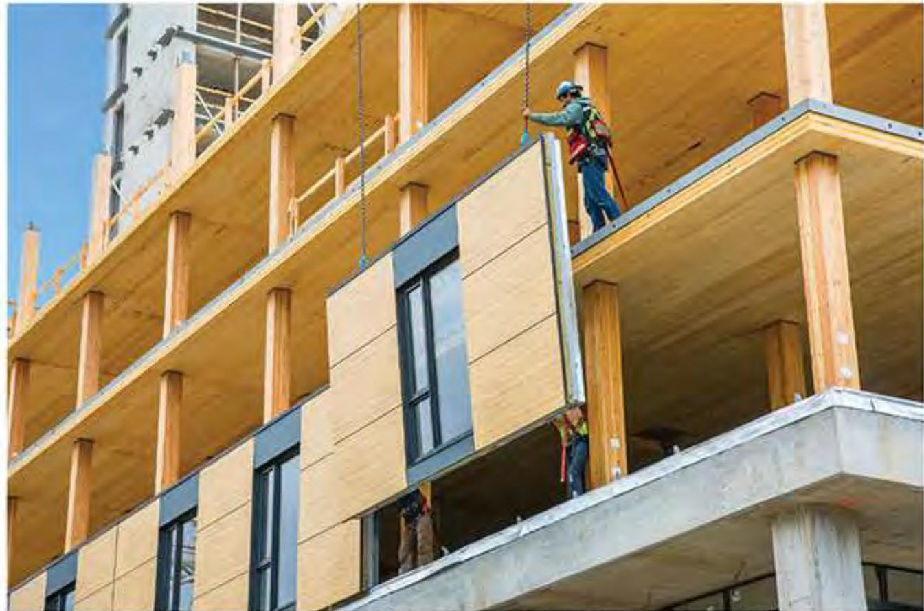
The prefabricated facade consists of steel stud framing with exterior sheathing, insulation and **Trespa® Meteon®** [distributed by **ATS-Sales**] for the rainscreen, attached with fibreglass '**Cascadia Clips**' which significantly reduce thermal bridging compared to a more traditional metal girt cladding system.
